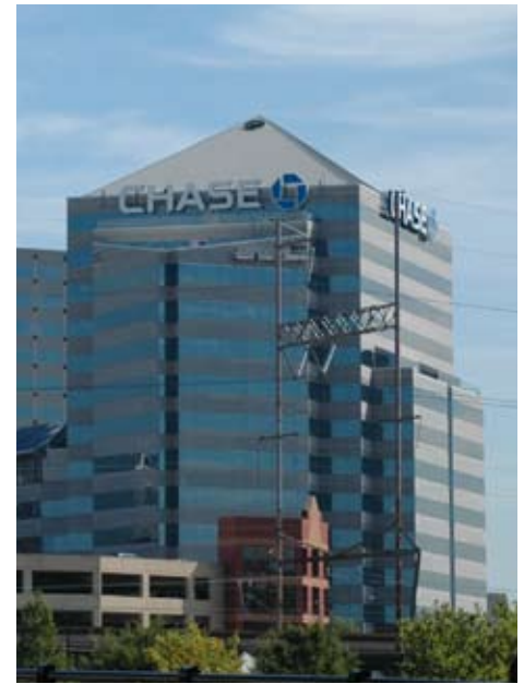
Chase building, Wilmington
